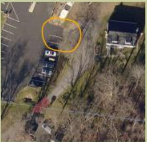
Image 2. An aerial view of the property highlighting access points during construction.
